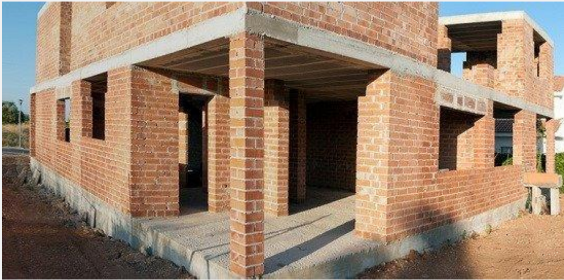
Fig: Load Bearing Masonry Wall
